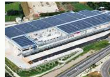
Courtesy of Shizuoka Branch of HAZAMA ANDO CORPORATION
